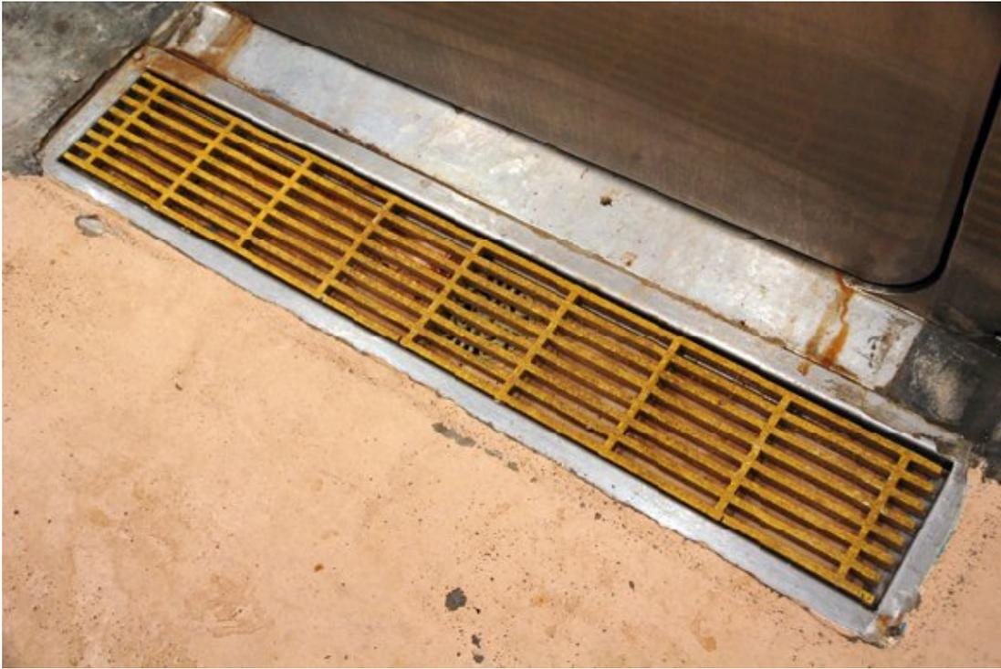
A drain at the entrance of a cooler doorway. The drain could become contaminated with *Lm*, and when employees step on the drain to enter the cooler, the *Lm* can spread into the cooler.
