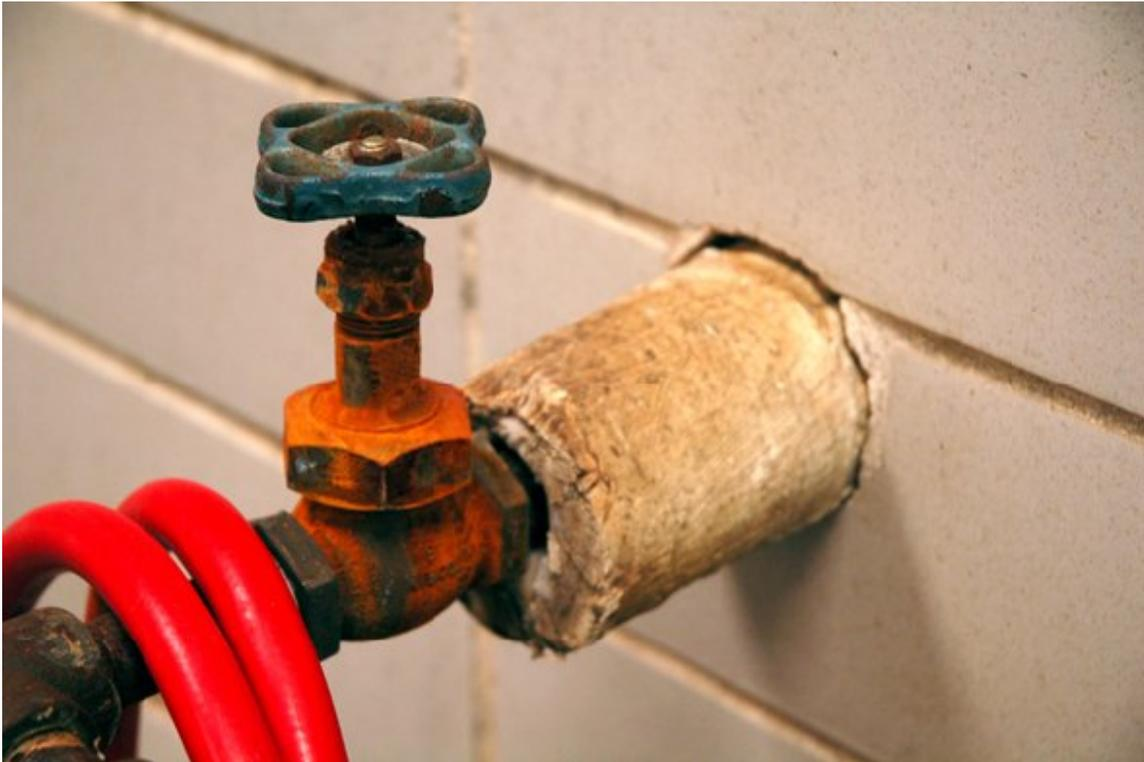
A rusty water spigot with a dirty, cracked insulated pipe. *Lm* could spread to the hose and be sprayed in the establishment.
